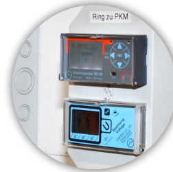
IKI-50 + CAPDIS (Directional Fault Detection)
