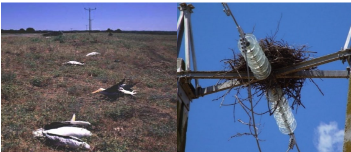
Figure 6. Pelicans dead from clashing conductors, Israel and nest likely to cause flashover, Spain.
