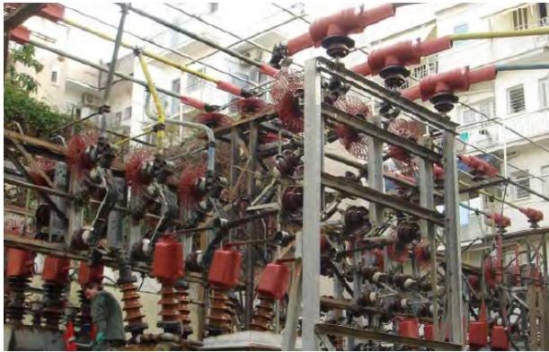
An ageing medium voltage substation in central Athens with huge numbers of cats and pigeons. Many phase to ground clearances well below the nominal 40cm distances and previously suffered multiple flashovers. Solution was to cover the vulnerable bare metalwork with a range of high performance polymeric covers, wraparound sleeving and circular barriers that prevent cats climbing over the insulator and being able to touch Medium Voltage and ground at the same time.
