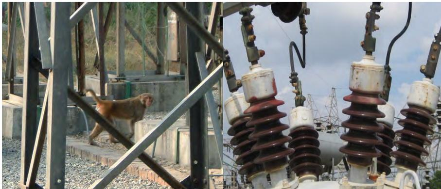
Figure 7. Monkeys in Indian substation and evidence of inter-phase bridging, Greece
