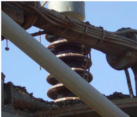
Figure 3. Guano build-up on suspension insulator and on substation equipment.
