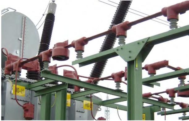
This substation in Croatia shows all bare live metalwork insulated, busbars with heat shrink tubing, connection points with cold applied wrap around covers that can be removed for maintenance or inspection and re-used. The issue was phase to ground clearances on medium voltage side of transformer and bus network where typical 40cm air gaps were being bridged by cats and birds (crows & pigeons).
