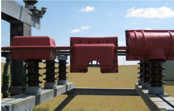
This 20 kV substation in rural Germany is insulated against climbing animals such as martens and cats using wraparound covers that are field cut on site to accommodate any unusual geometry including the center cover where a cut-out has been added to allow access for an earth clamp in a relatively safe position. Covers that need field cutting benefit from being produced from a polymeric cross linked material because they will never propagate splits if they are roughly cut.
