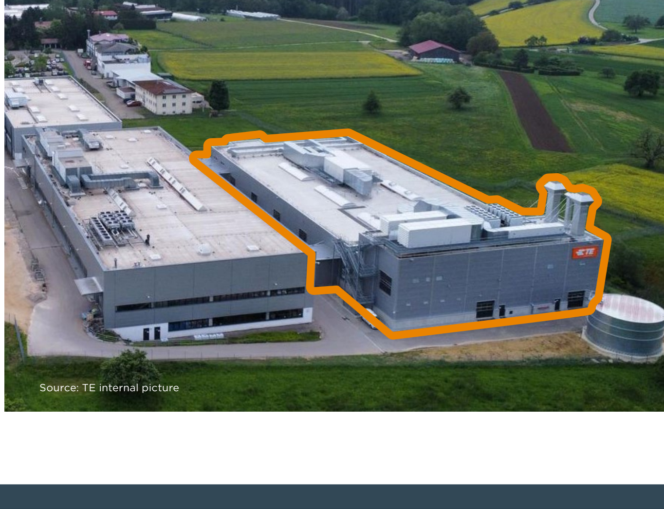
TE Plating shop, Germany
