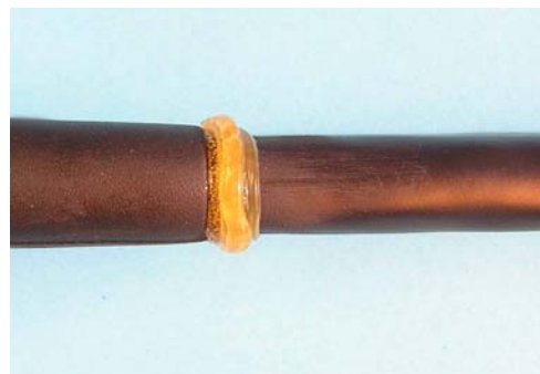
NOT ACCEPTABLE Excess adhesive flow /42, /86
