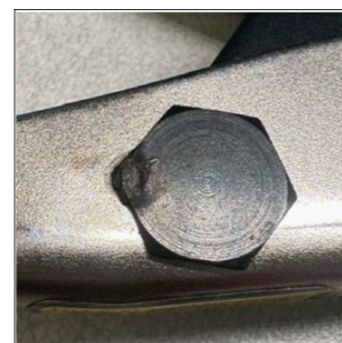
TAC WELDING CAM ADJUSTMENT SCREW TO FRAME AFTER VERIFICATION PER NOTE 4 IS AN ACCEPTED OPTION.
