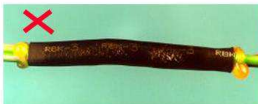
2. Overheat of tubing
