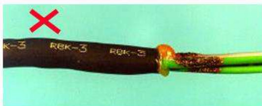
3. Overheat of wires
