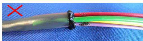
3. Overheat of wires
