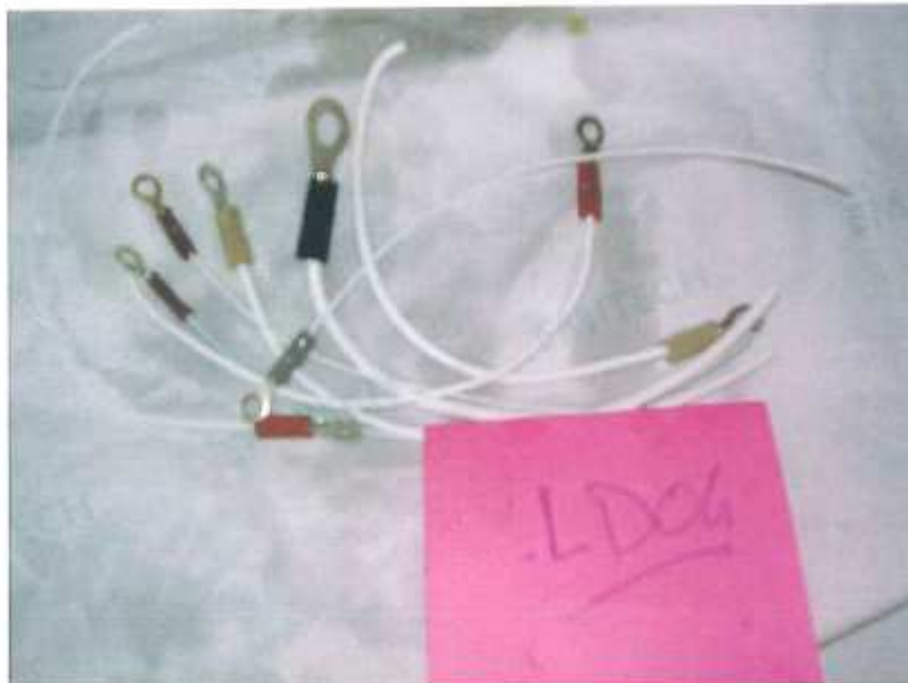
Photography of the equipment after tests LD04
