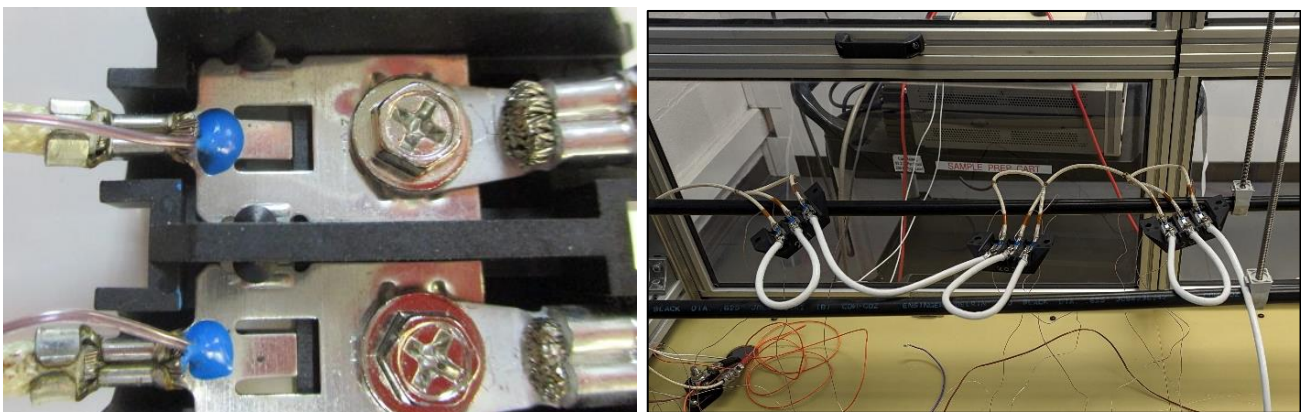
Figure 6 – Thermocouple Location and Typical T-Rise Test Setup
