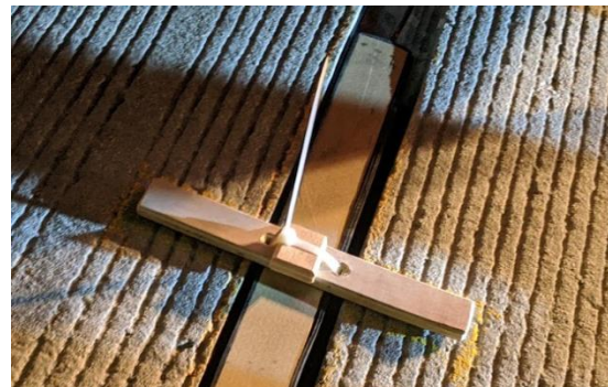
Figure 6. Attachment and Use of Mounting Brackets
