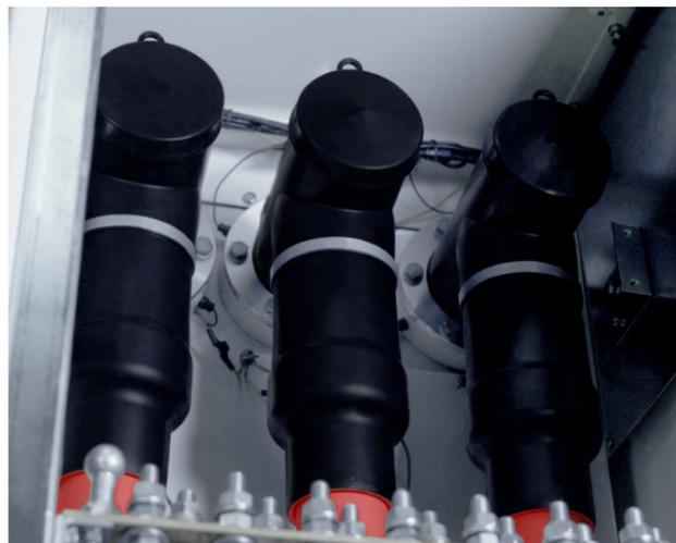
RAYCHEM RSTF CONNECTORS ARE ALSO COMPATIBLE WITH SIEMENS ENERGY BLUE GIS WITH CLEAN AIR
