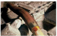
After the joint area has been smoothed out with strips of electrical filler, the adhesive-coated outer sleeve is shrunk into place to restore the cable oversheath and complete the joint.
