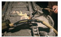
Flexible heat-shrinkable sleeves are first slipped over the cable core ends and the conductors jointed. The sleeves are then shrunk down over the connectors to insulate them and seal out fluids and chemicals.
