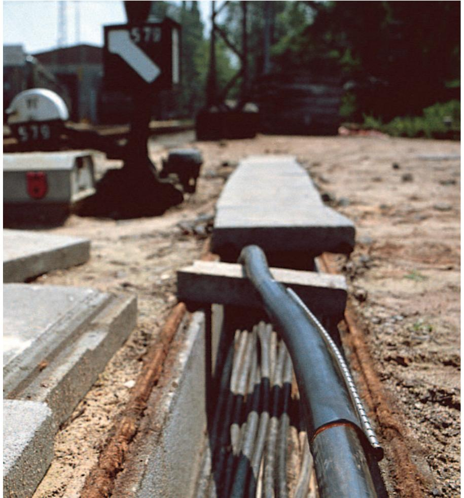
CRSM wraparounds are used in a railway goods yard in Germany to restore the insulating, sealing and mechanical protection functions of damaged cable oversheaths.
