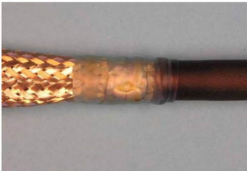
NOT ACCEPTABLE Insufficient solder flow
