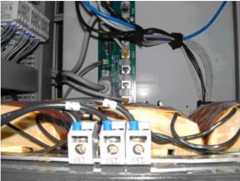
Figure 166 — T2 Secondary Terminals
