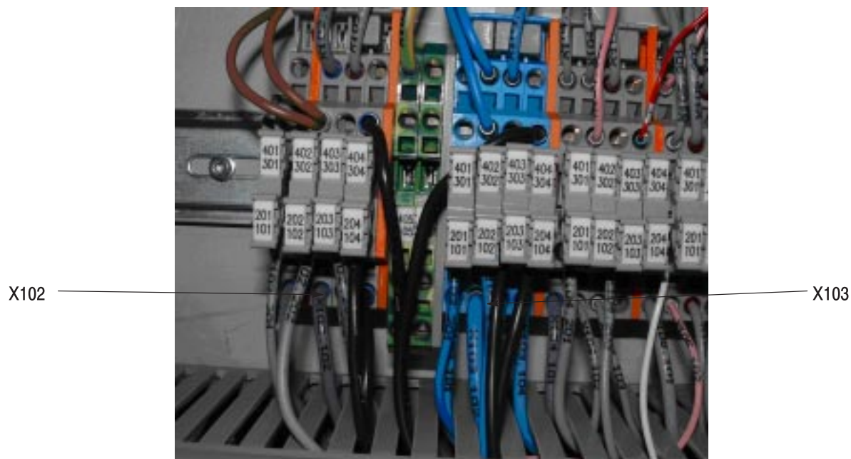
ST III Control Power Connection Internal to AMPOMATOR System III Control Cabinet (Center)
