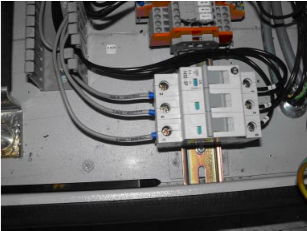
Wiring and Mounting for CB-1 Positions 2, 4, and 6
